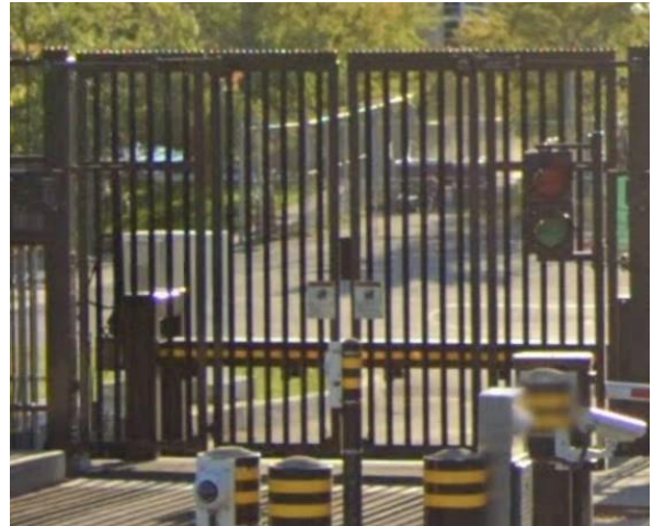
Panel fabric fence and gate with vehicle security barrier and external bollards. Figure 2
