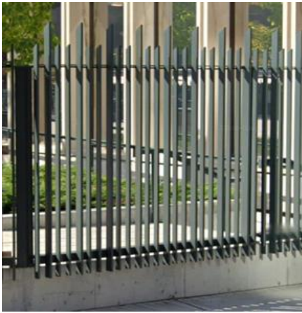
Panel fabric with deep vertical bars and concrete extended base
