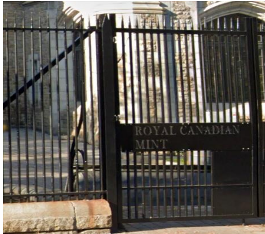
Panel fabric with narrow vertical poles, extended base, and vehicle stop behind the gate. Figure 1
