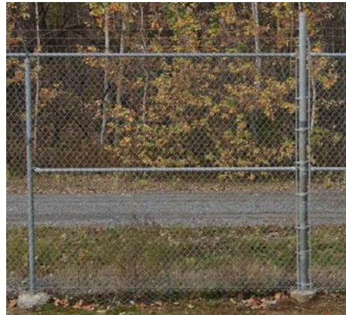
3-wire barbed wire installation with twist end fabric and strain post
